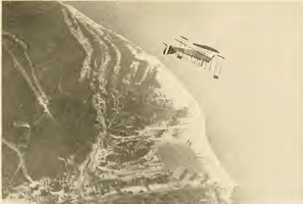
SPIRALLING AN N-10 ON ITS BACK AT PENSACOLA
