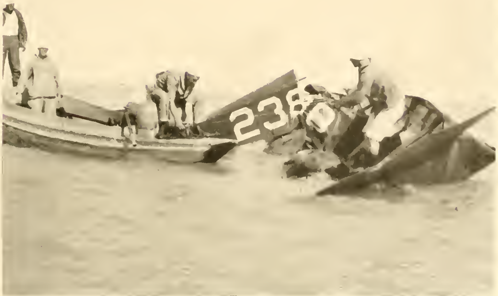
ANOTHER JOB FOR THE WRECKING CREW
